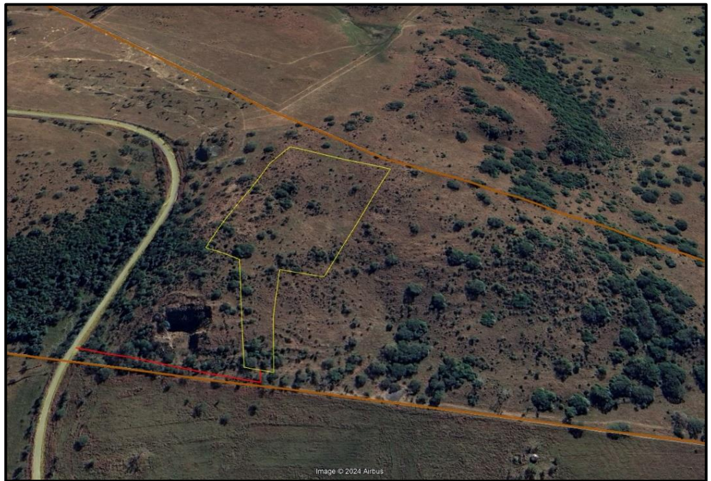
Figure 3: Satellite view showing the path of the existing access road (red line) to the proposed mining area (yellow polygon).
